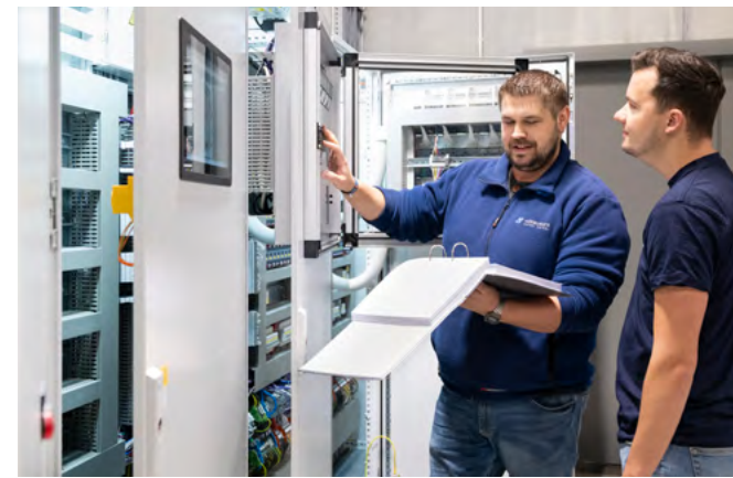
Martin Hartmann (Project Manager, Hörburger GmbH, left), Dominik Gruber (Commissioning Technician, Hörburger GmbH)
