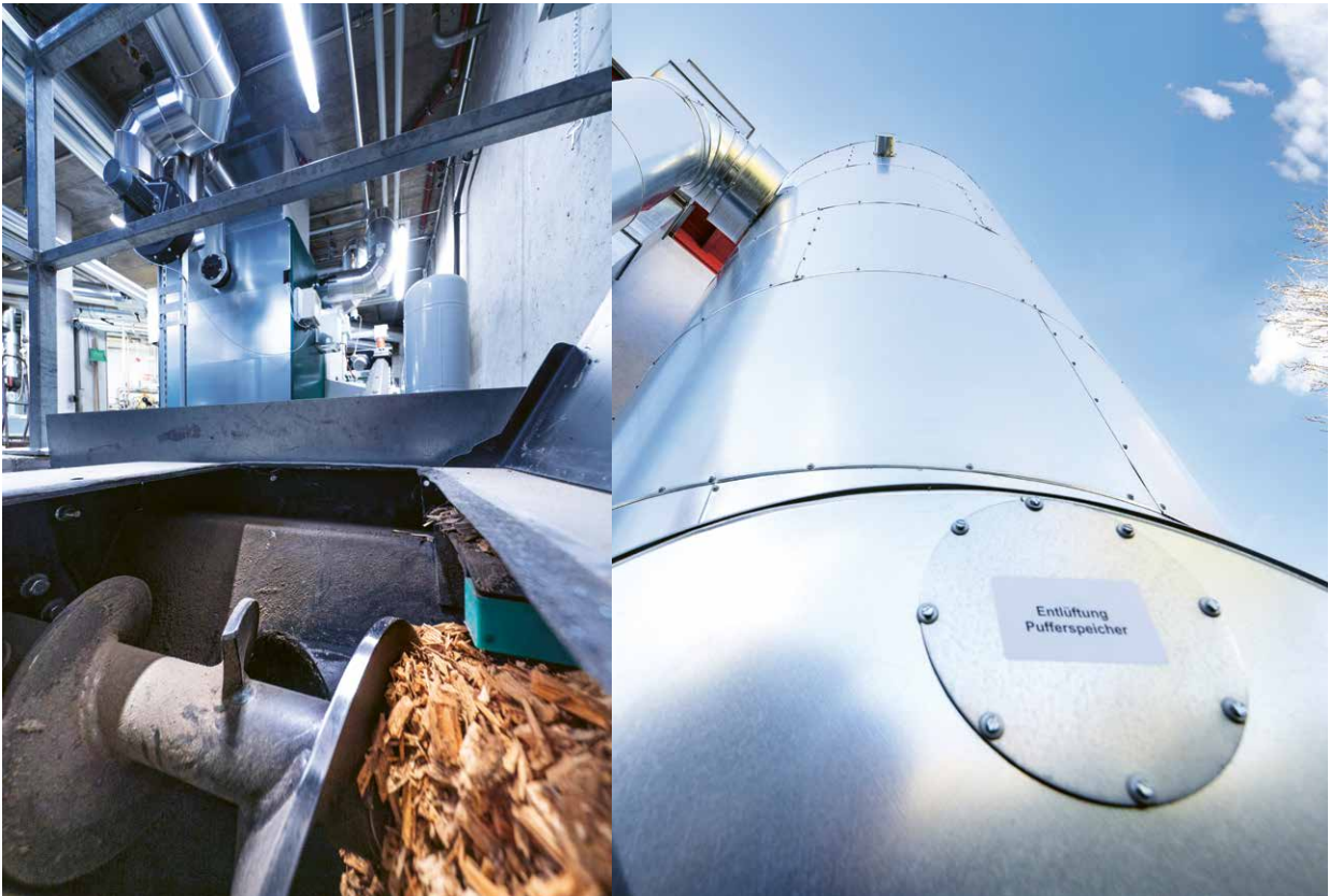
The new storage tank was set up outdoors and has a capacity of 20,000 liters of hot water, creating room for a larger wood-fired boiler in the central heating system.
