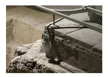
And third, the security system was to remain discrete without interfering with the experience of the life-sized warrior and horse figures. Keeping these factors in mind, Bosch experts deployed a combination of several hundred intrusion detectors across the 16,300-square-meter museum area. For rapid detection of security breaches, the team installed wall-mounted detectors in the pits alongside the clay warriors, supplemented by ceiling-mounted detectors above visitor walkways and open areas.
