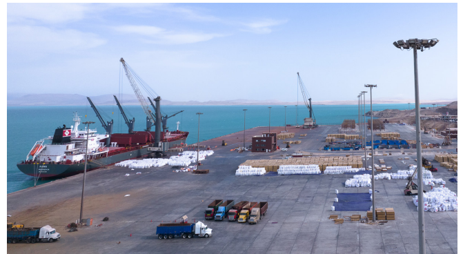
Terminal Porto Paracas
