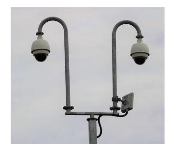
All cameras with starlight technology continue to deliver full intelligent analytics at night and in low light levels. The cameras installed around the depots are able to provide colour filtering down to 0.0077 lux or deliver detailed monochrome images where other cameras show no image at all.
