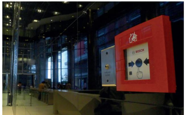
Panel 5000 Series. At Citibank Plaza, the solution is also part of the Bosch Building Integration System (BIS). This integration allows operators to use the BIS Automation Engine as the graphical user interface (GUI) for monitoring and control of alarms.
