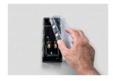
**2. PROTECT**Apply the paint cover to protect the wall-mount until construction is completed
